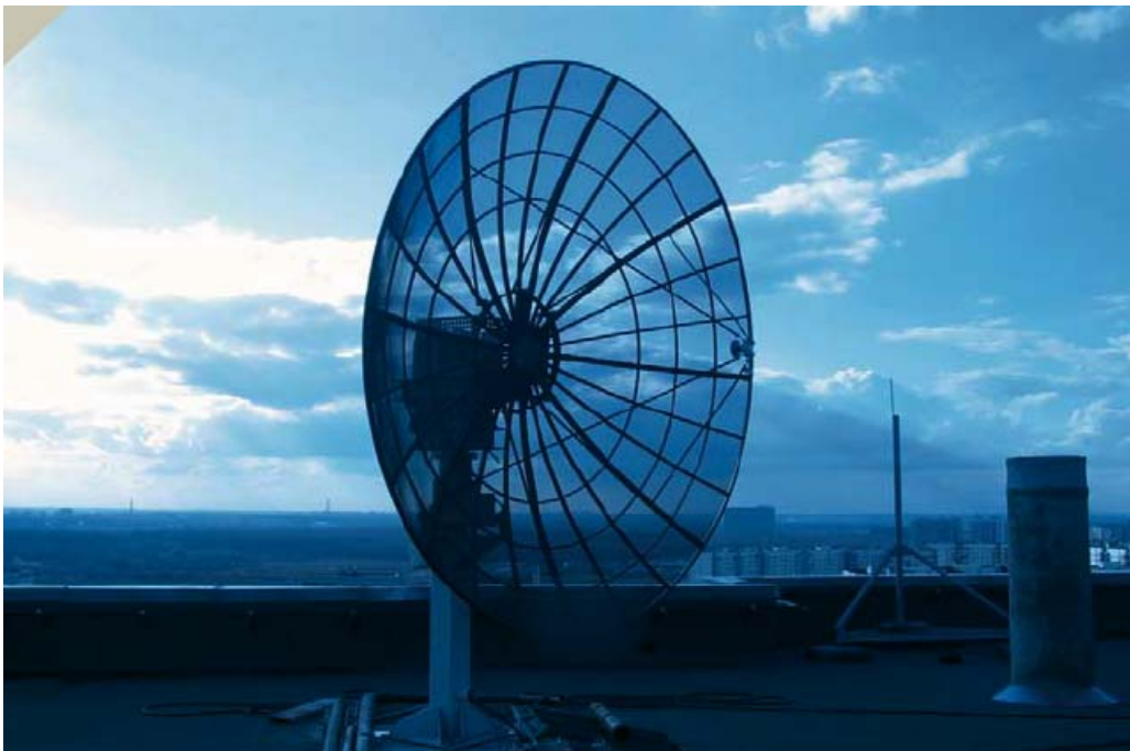
UniScan-36 ground station with the 3.6 m antenna installed in the Moscow Center for data reception and processing of ScanEx R&D Center. Nowadays it is the most universal domestic complex, providing for the data reception from 11 satellites of the leading RS operators in the USA, India, Israel, France, European space agency, Russia and Canada.
